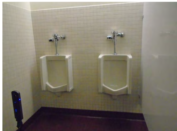
Fig. P-12 – Typical wall mounted side-by-side urinals
