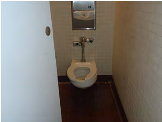
Fig. P-1 – Typical Wall Mounted Water Closet
