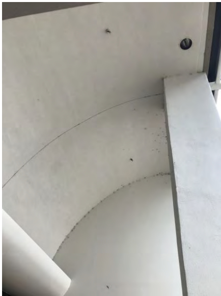
Fig. F-5 – Dry pipe sprinkler heads at front canopy entry
