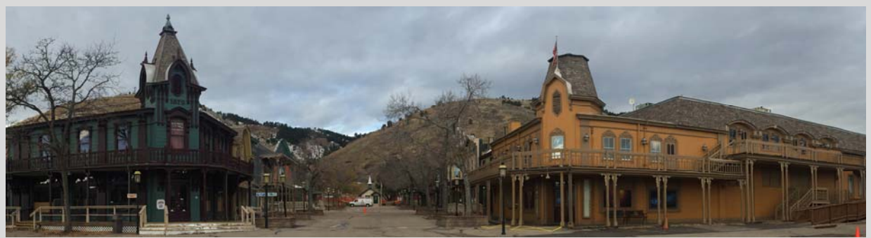
Building A on the left and Building D on the right frame the entrance plaza and the main street
