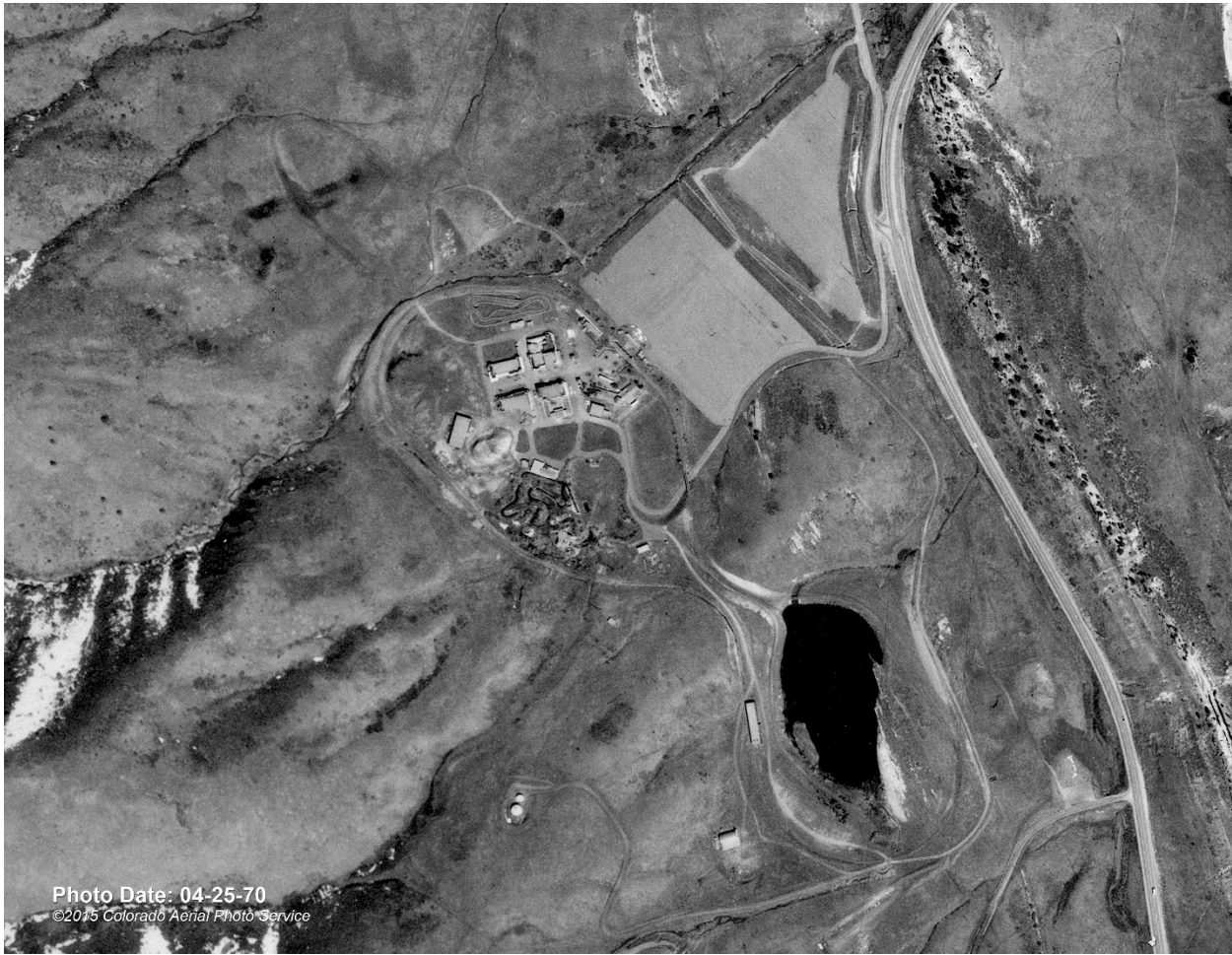
1970 This photo was taken toward the end of the dormant period of Heritage Square. No visible differences in buildings are evident in this photo. Note that the lake in the amusement park area appears dry. No cars are visible in the parking lot.
