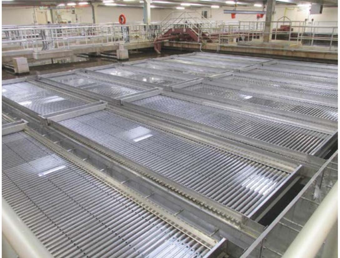
methods. Previously, solids were removed primarily using gravity; a slow process rarely used in modern water treatment. With the addition of plate settlers, solids are removed more efficiently.
