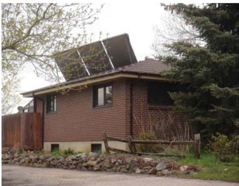
These roof-mounted solar panels are rotated due south. It is preferable to keep panels closer to the roof surface for aesthetic reasons.
