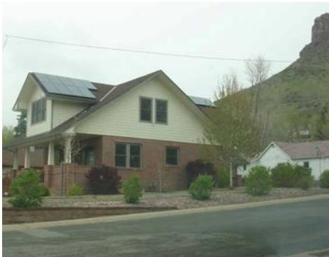
While this is a good effort to provide on-site power, these photovoltaic panels are facing 35 degrees east of south per the Golden grid, and the limited number of panels would not provide a net-zero installation.
