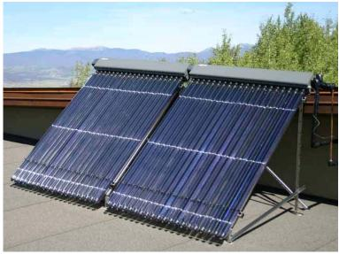
Evacuated tube solar hot water collectors
